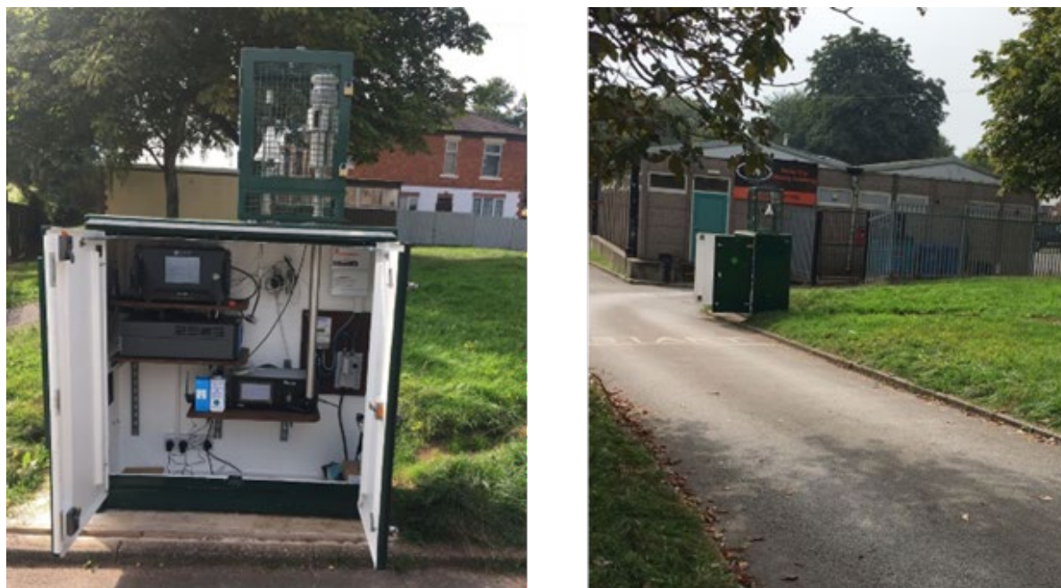
Figure 2 – PR5 housing at Derby Stockbrook Park site.
