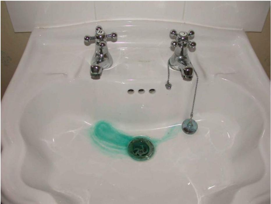
**Figure 5.** (a) Irregular carbonate patina giving rise to blue water; (b) Staining in hand basin caused by blue water.
