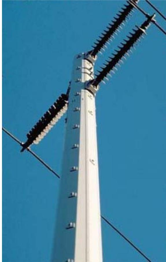
**Figure 1 Composite distribution pole (courtesy of Strongwell Corporation)**
