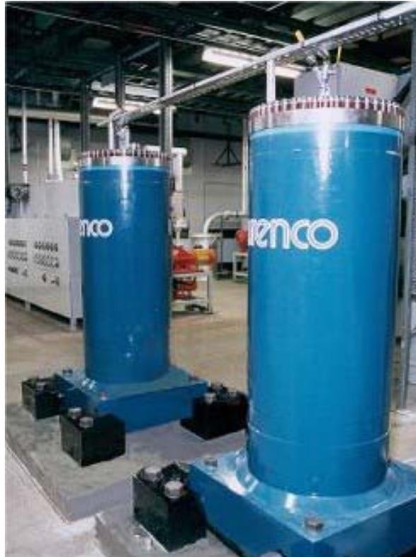
**Figure 7 PQ Series flywheel installed at Urenco's plant in Cheshire
